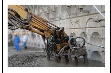
Optional rotating head allowing vibrator assembly to work in restricted space as well as closely against existing structures. Labor reduction is significant, saving time and reducing cost.
